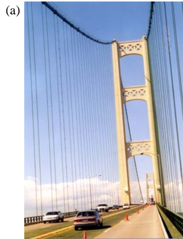
Cables of Mackinaw bridge
